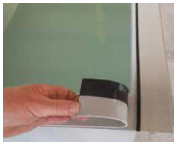
When applying sealant to the next flange, ensure a overlap.
