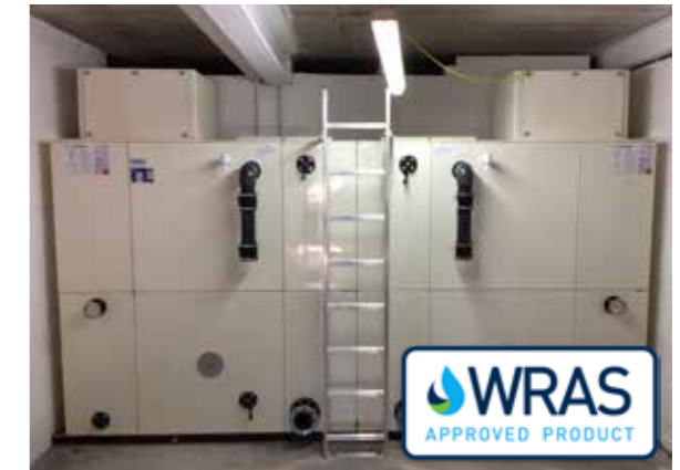
TIF tank - totally internally flanged option shown
